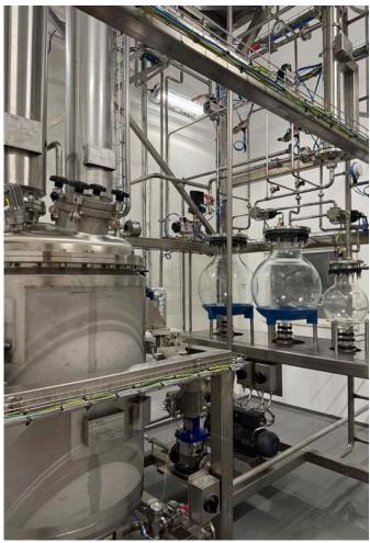
**Fractional distillation and rectification** – The final stage of the process involves fractional distillation in glass collection chambers. This allows for separation of specific compounds such as d-carvone and d-limonene, ensuring consistency and high purity for specialised end uses.
