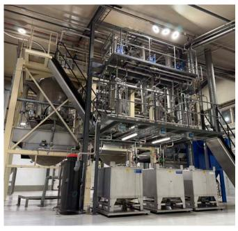
Cooling and condensation system – The separation unit located adjacent to the distillers features a two-stage cooling system. Vapours first pass through a primary condenser and then a heat exchanger, enabling recovery and reuse of approximately 15% of the thermal energy.
