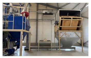
Seed intake, feed system, and top of distillers – Seeds are delivered in large containers or bulk bags and transferred into the feed unit. From there, a pneumatic system conveys the material through stainless-steel pipes directly into the distillers, located in a separate section of the facility. At the upper level, the feed system ensures the continuous transfer of seeds into the distillers for steam distillation.
