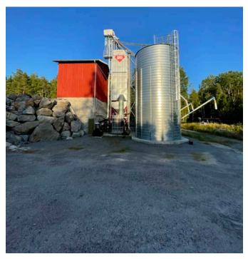
Farmers unload caraway at the red unloading bay before it enters the central dryer, where warm air dries the crop and cool air prepares it for storage.
